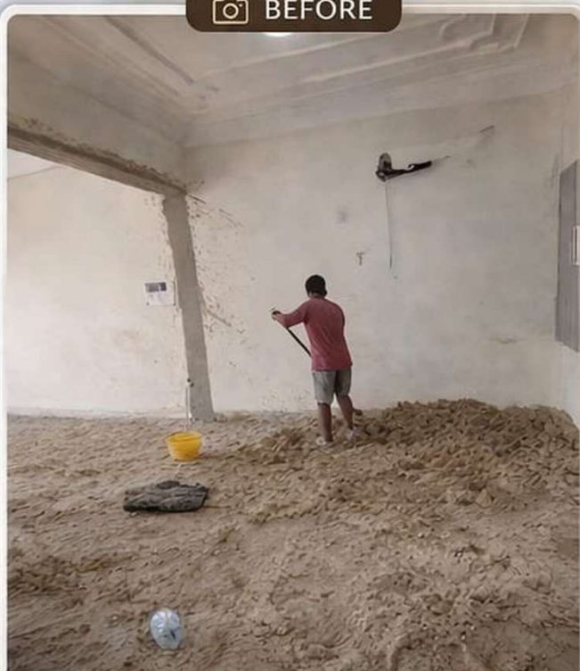
Initial site condition — Structural stage
